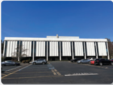
Starux, Inc. Headquarters in New Jersey
